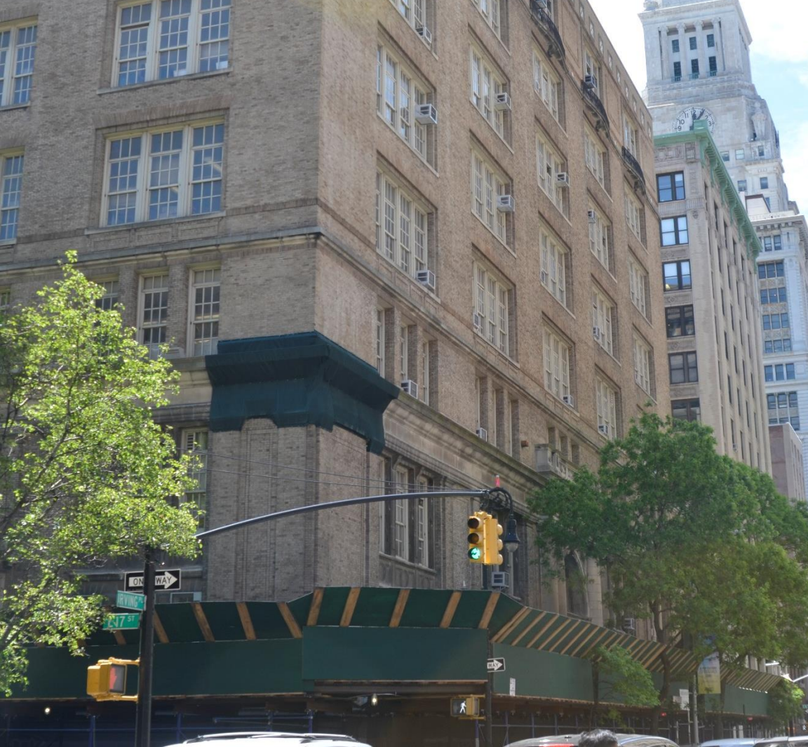
Netting at the northwest corner of the cornice and Sidewalk Sheds surrounding the facades
