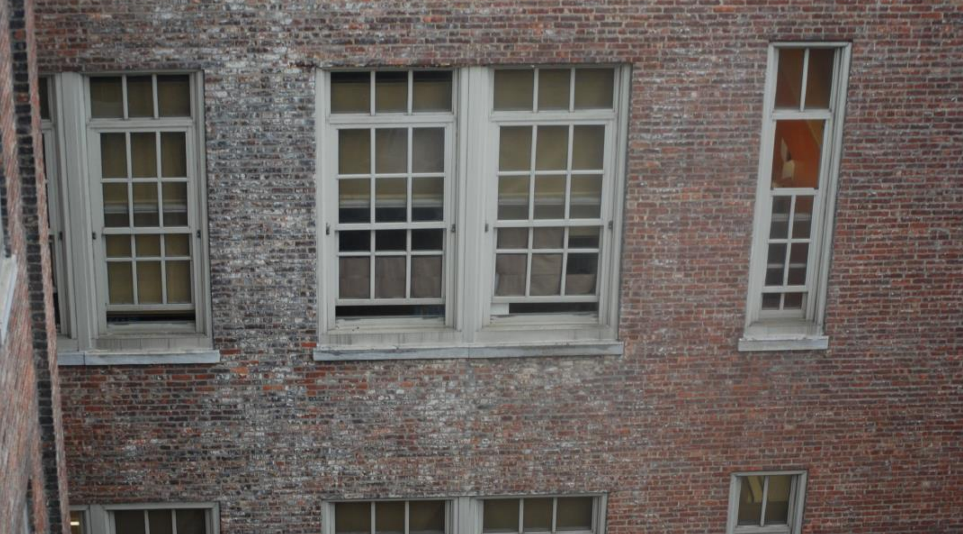
Photo 377: Original Building, North Court Elevation
