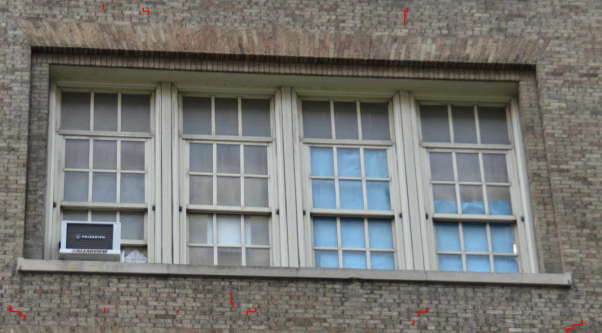
Original Building West façade, 5 th floor
