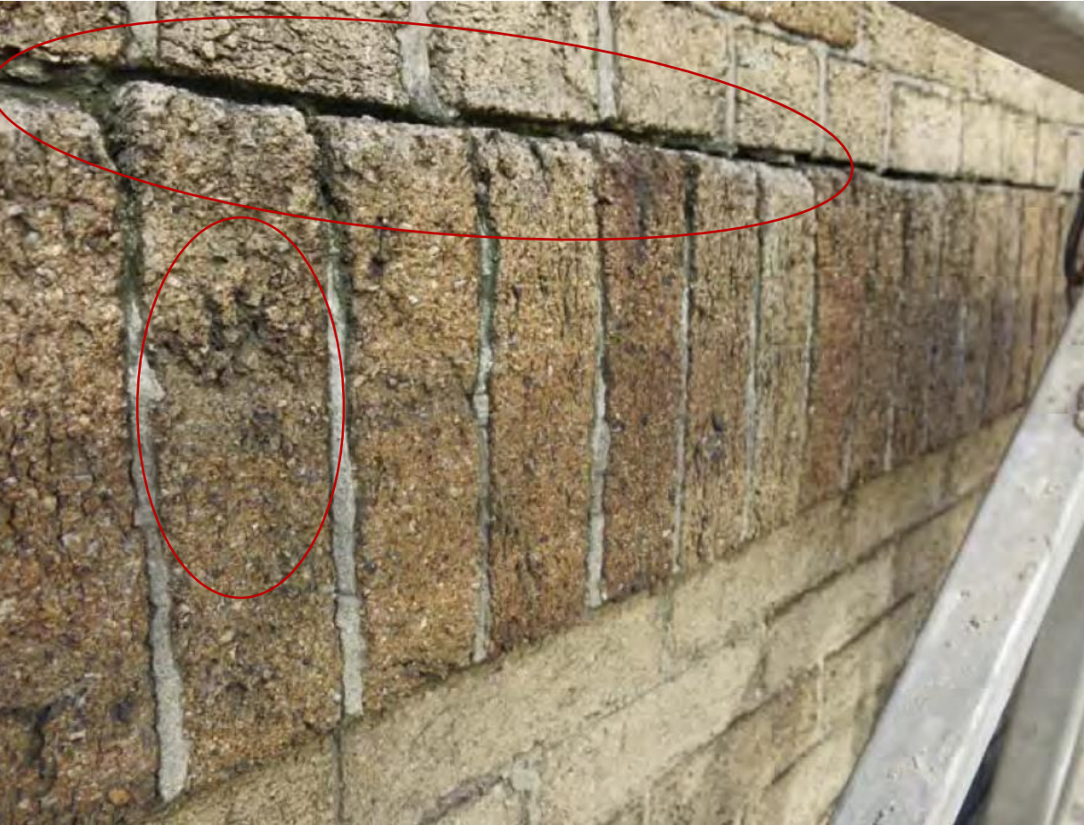
Drop Location # 1 – West Elevation; fourth floor
