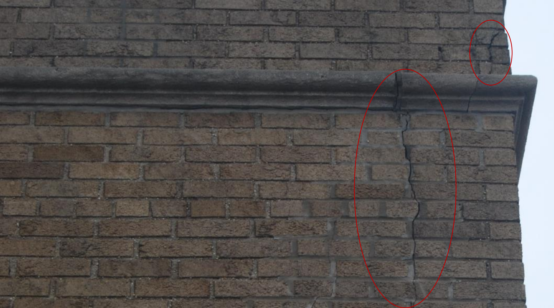
Photo 386: Additional Building Bulkhead, northeast corner
