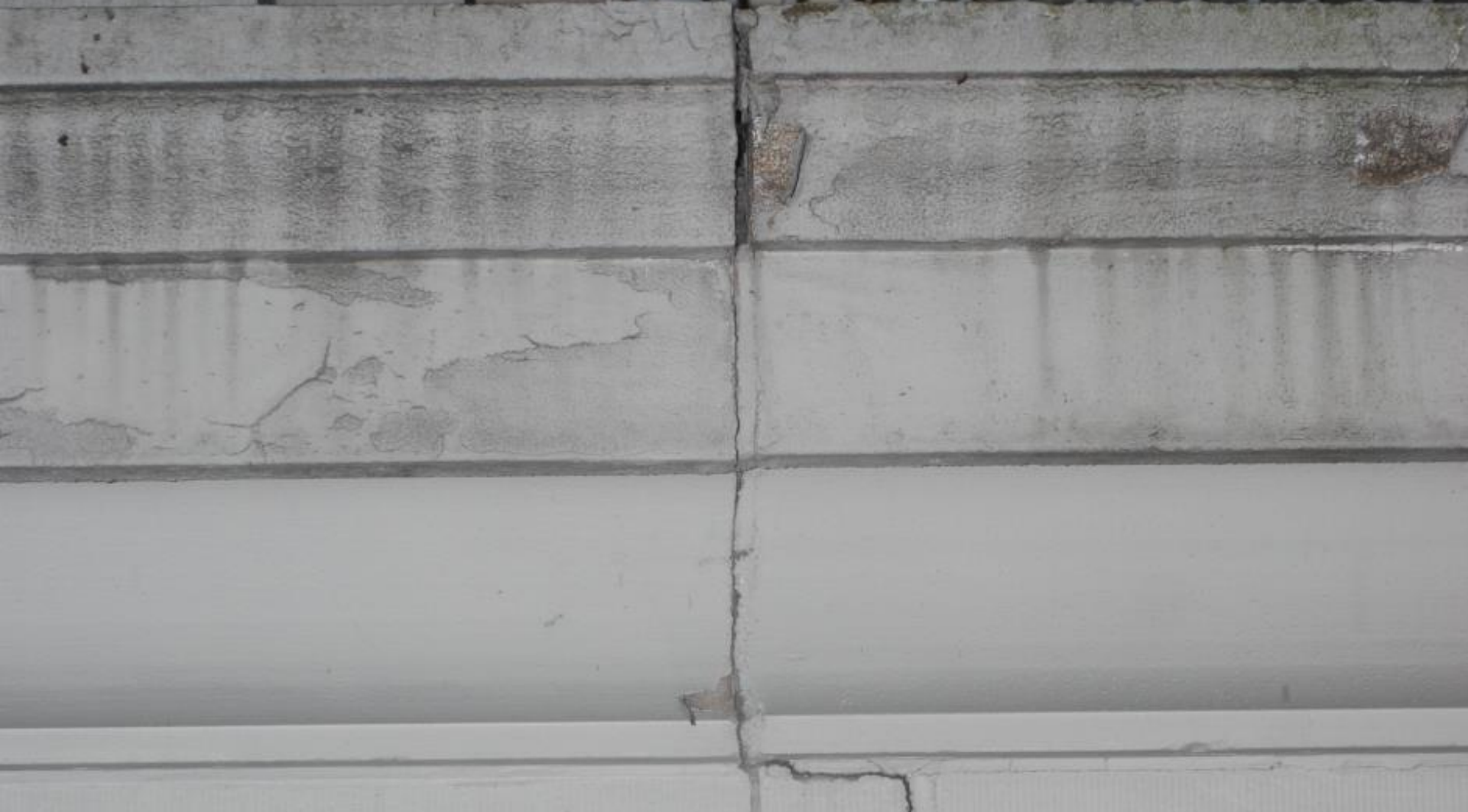
Photo 354: Original Building West façade, first floor
