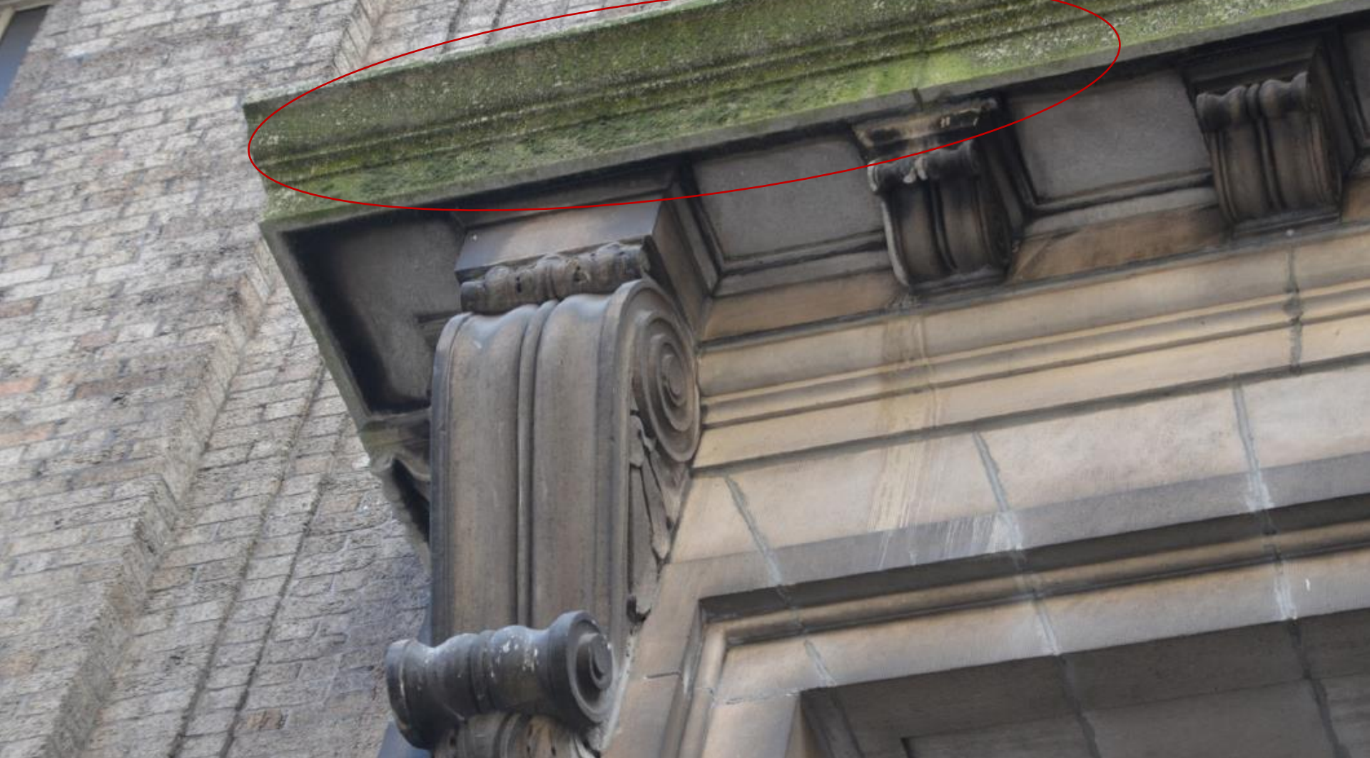
Photo 365: Original Building, North facade
