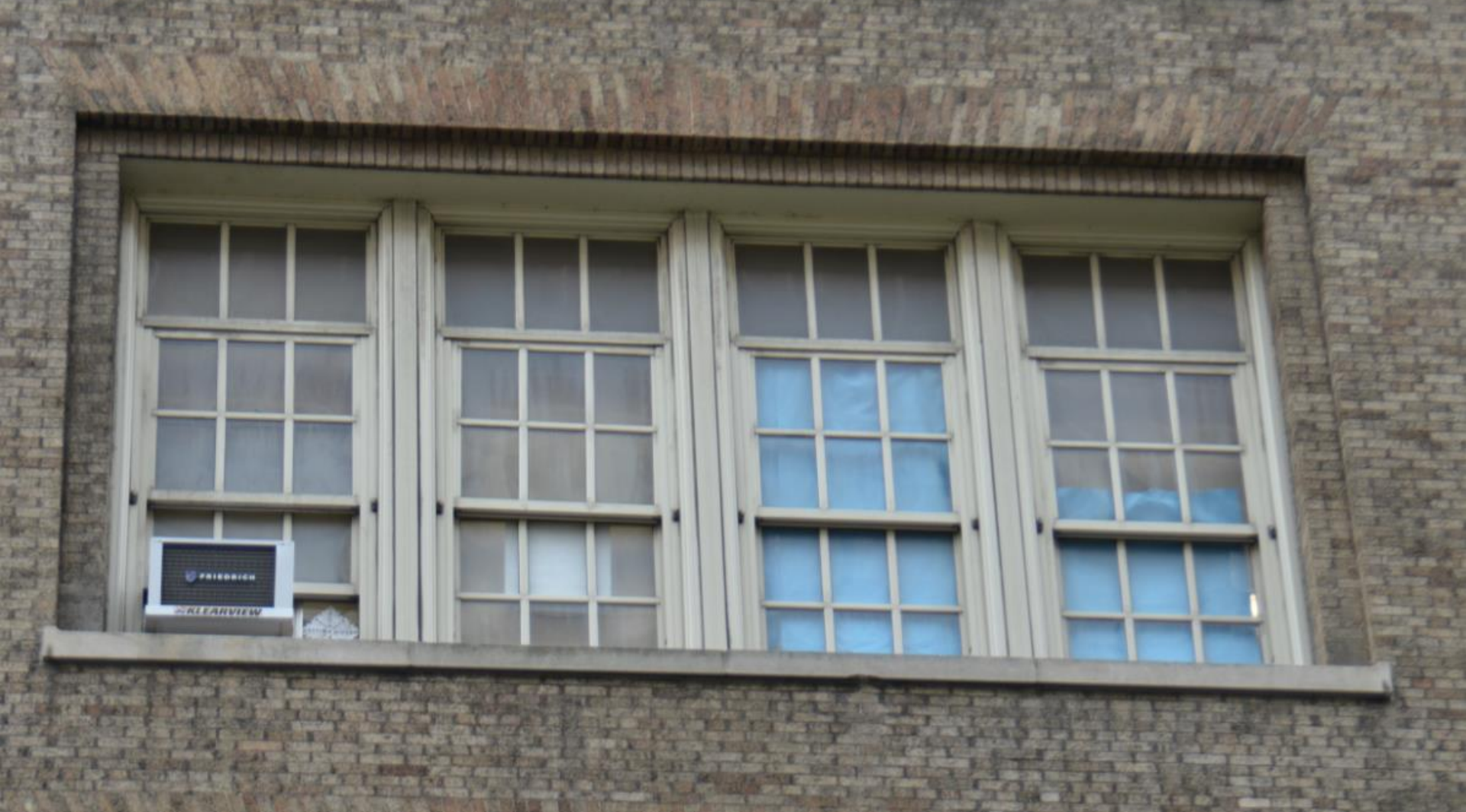
Original Building West façade, 5 th floor
