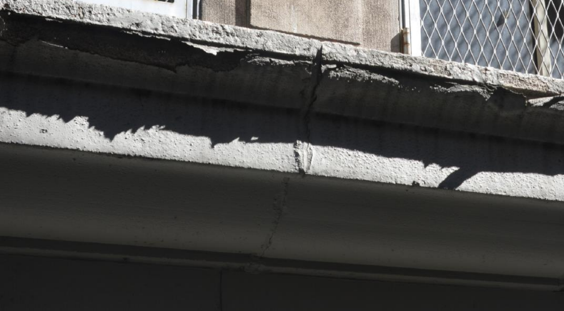
Photo 343: Original Building West façade
