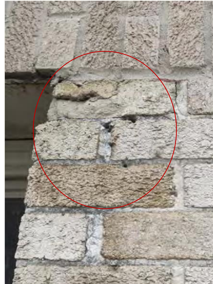
Drop Location # 2 – South Elevation; eighth floor
