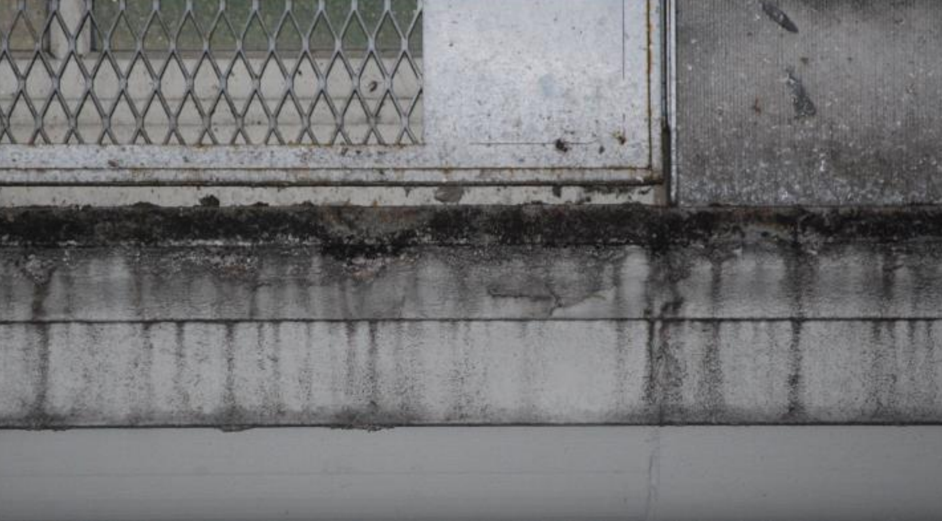
Photo 355: Original Building West façade, 1 st floor
