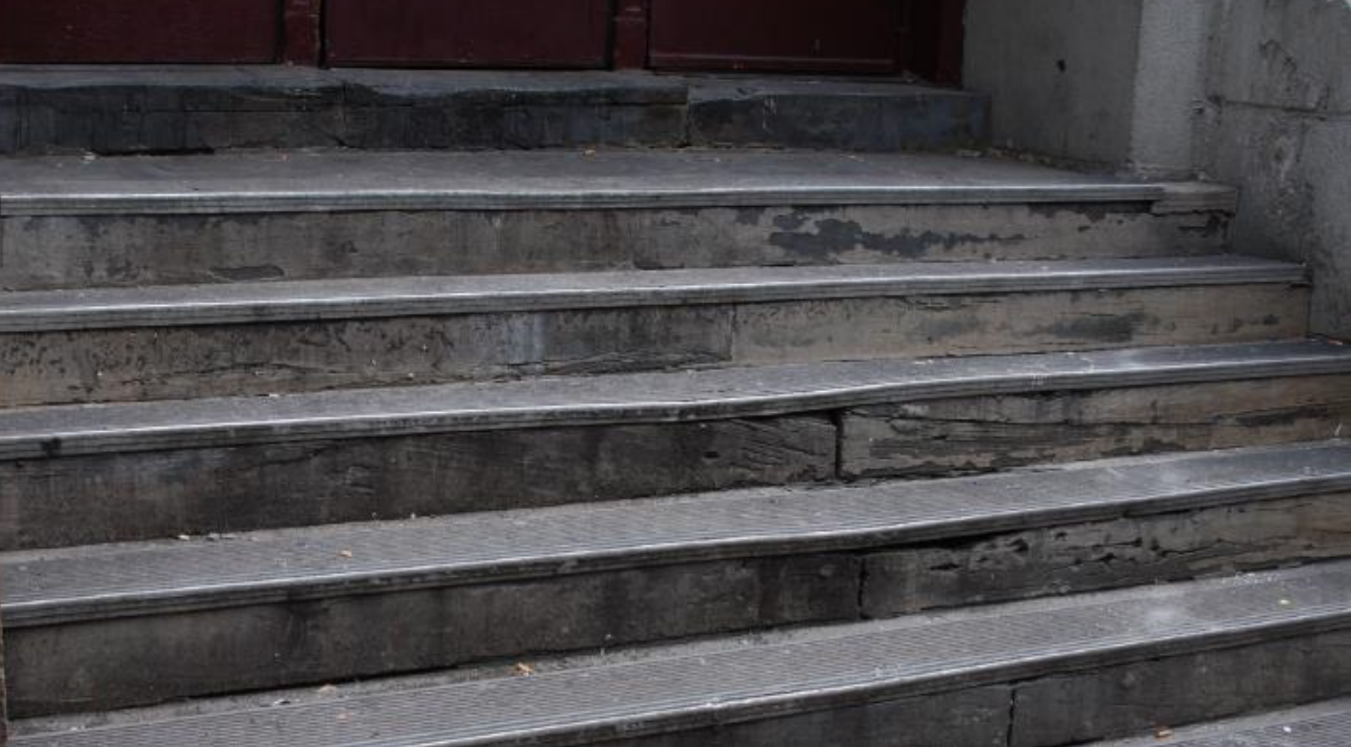
Photo 325: Original Building South facade
