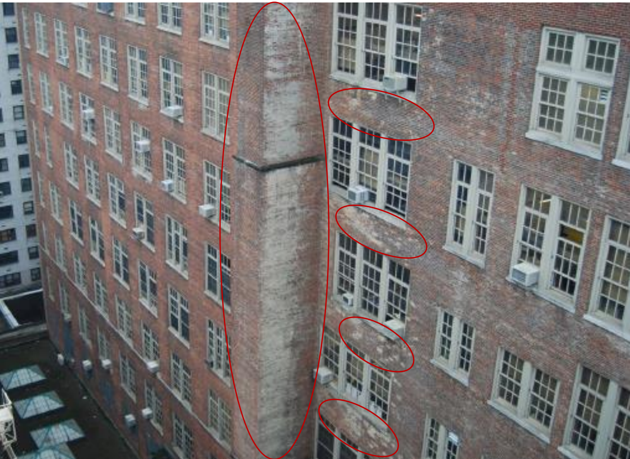
Original and Additional Building, South Court Facade
