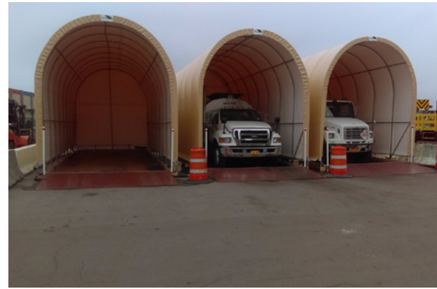
DOT trucks under cover and within secondary containment
