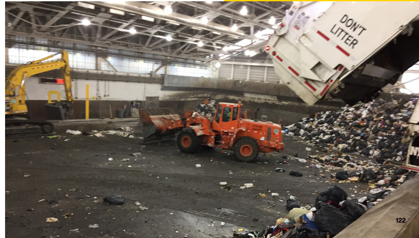
DSNY fully-enclosed marine transfer station
