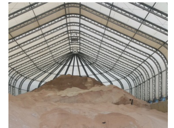
DSNY salt shed
