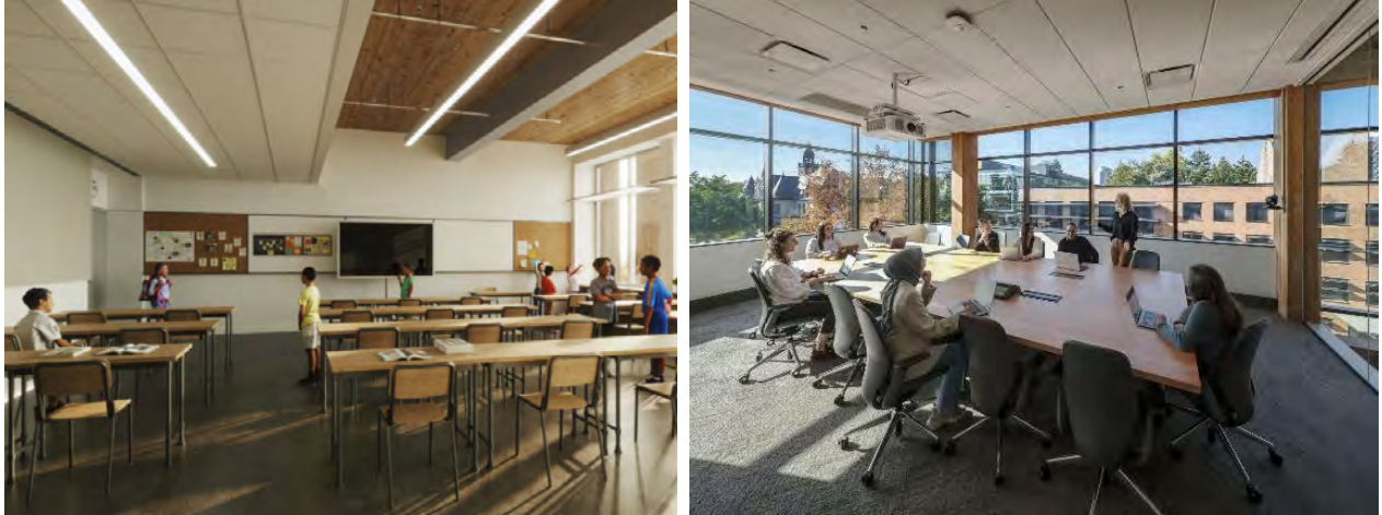
Figure 37. Dropped Ceilings at Evergreen Charter School, Hempstead, NY (left, Martin Hopp Architects) and Founders Hall, University of Washington, Seattle, WA (right, LMN Architects)
