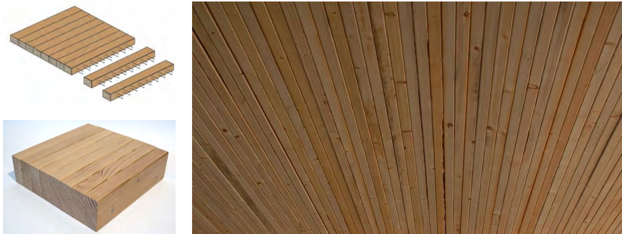
Figure 6. Nail-Laminated Timber: Diagram (top left, Abed et al., 2022); Sample of Prefabricated NLT Panel (bottom left, naturallywood.com); Site-Fabricated NLT Floor Plate (right, StructureCraft)
