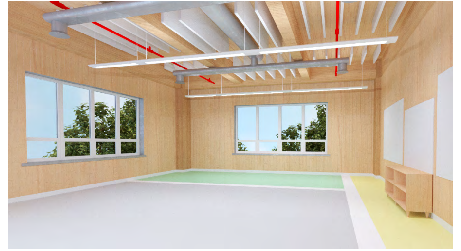
Figure 86. Fully Exposed CLT Ceiling with Acoustic Baffles
