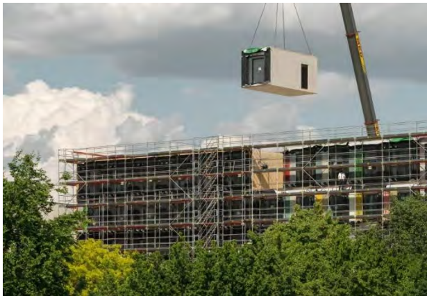
Figure 40. Fully Modular MT Construction: “Luisenblock” Parliamentary Office Building, Berlin, Germany (left, Sauerbruch Hutton Architects); Residential Modular MT Concept (right, Peter Rose + Partners)
