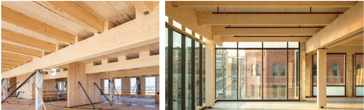
Figure 35. Stacked Beams at Catalyst, Spokane, WA (left, Michael Green Architecture/Katerra) and Platte 15, Denver, CO (right, OZ Architecture)
