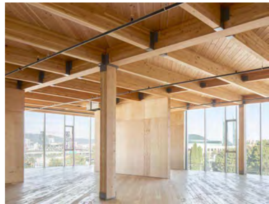
Figure 14. Post and Beam System (left: canadianarchitect.com; right: Joshua Jay Elliot)
