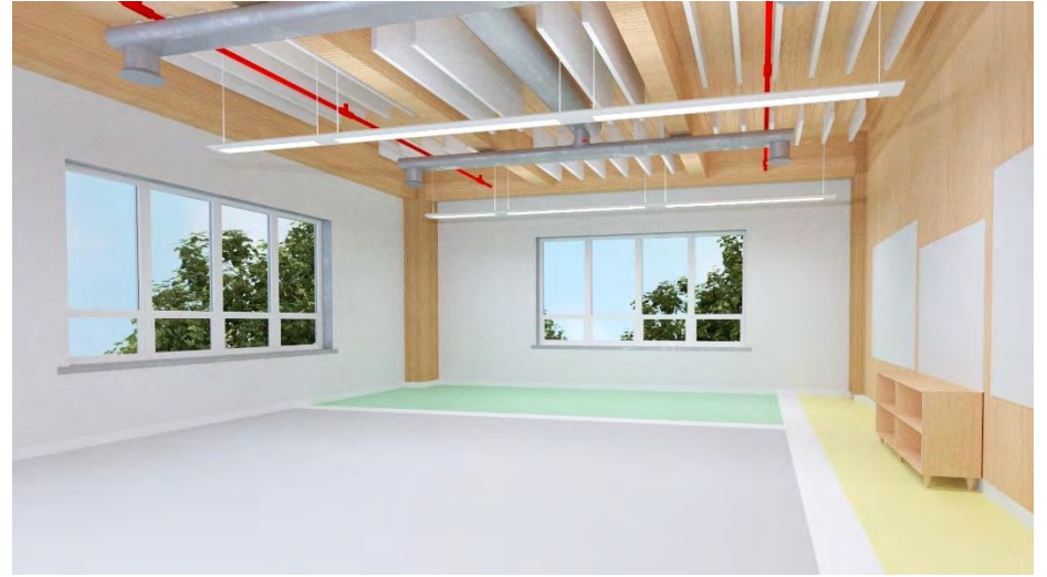
Figure 84. Fully Exposed CLT Ceiling with Acoustic Baffles
