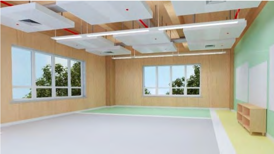
Figure 85. Partly Exposed CLT Ceiling with Integrated Ceiling Clouds
