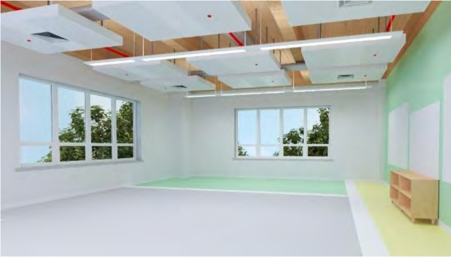
Figure 83. Partly Exposed CLT Ceiling with Integrated Ceiling Clouds
