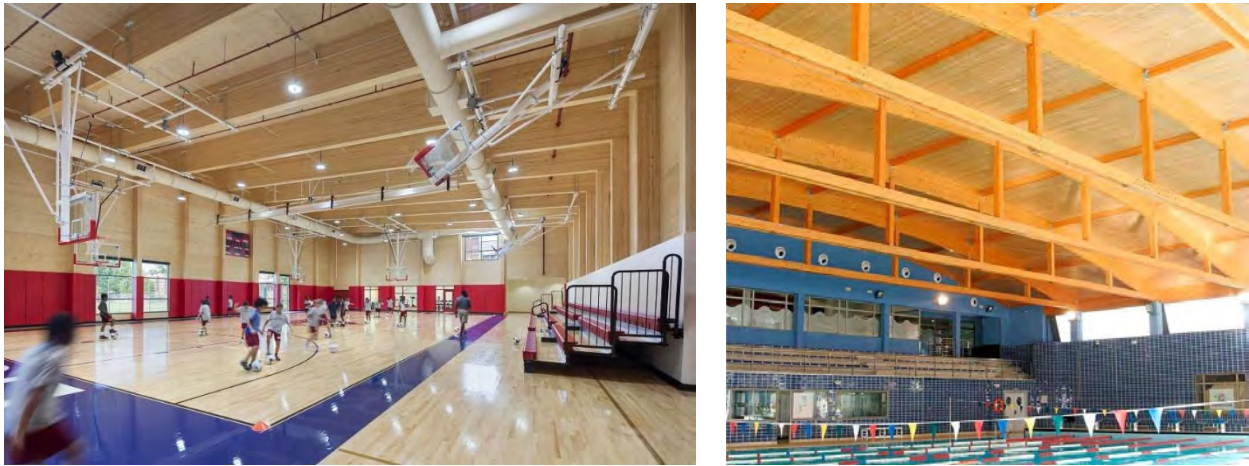
Figure 18. Long Span Systems Left: Simple deep GLT bents. Right: GLT bowstring truss and barrel roof. (left: ThinkWood; right: Kate Simonin)
