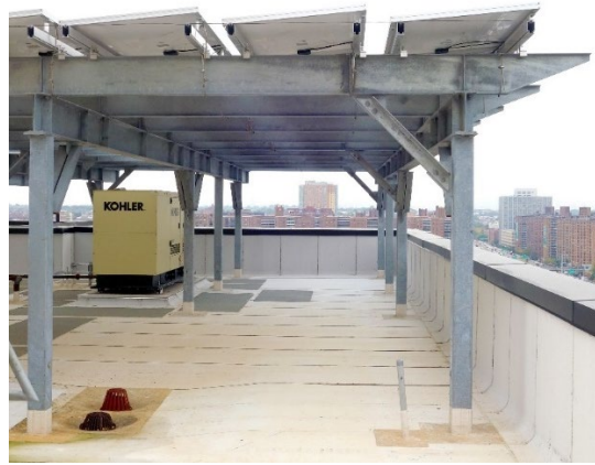
Building-aligned “sawtooth” PV canopy with 5° tilt angle at Apex Place, Queens (credit: FXCollaborative)
