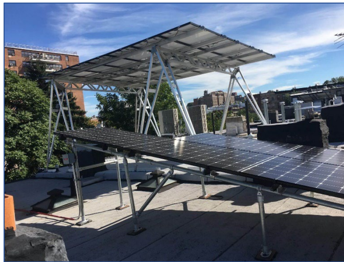
Brooklyn SolarWorks Canopy (rear) and Tilt Rack (foreground) PV Arrays
