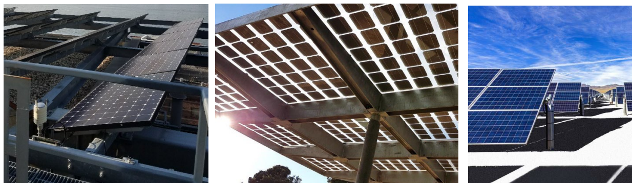
PV panel types, from left to right: solid monofacial, semi-transparent monofacial, and bi-facial (credits, from left to right: EME Group, www.onyxsolar.com , www.solarsena.com )
