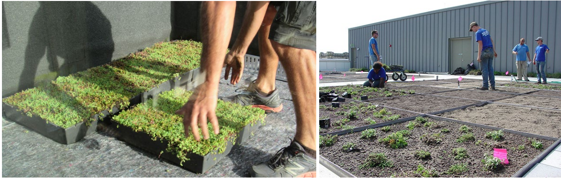
Illustrations of Modular (left) and Built-in-Place (right) Green Roof Systems (credit: www.wallbarn.com , Kansas State University Architecture, Planning, and Design)
