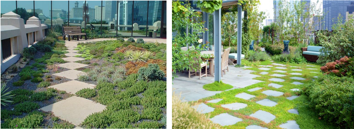
Pavers embedded in a modular green roof at Atlanta City Hall (left, credit: Waterproof! Magazine) and in a built-in-place intensive green roof in Battery Park City, NY (right, credit: MKM Landscape Architecture)
