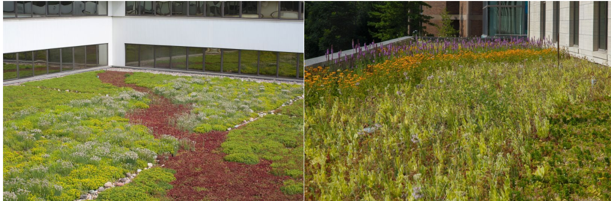
Illustrations of 4" Substrate with Sedum (left) and 6" Substrate with Mixed Grasses (right) (credit: www.liveroof.com )
