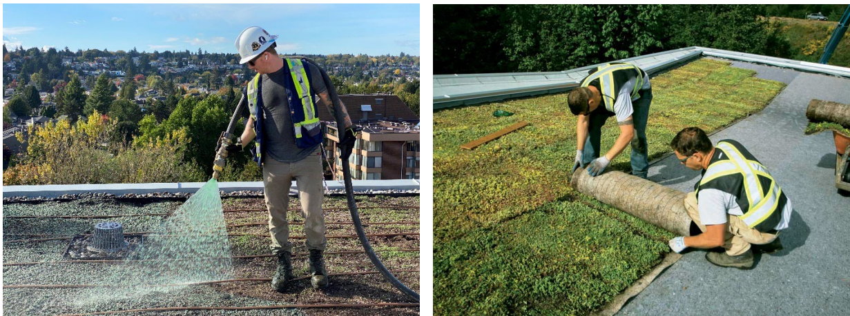
Illustrations of Grown in Place (left) and Pre-Grown Mat (right) Vegetation (credit: www.architek.com , www.constructioncanada.net )
