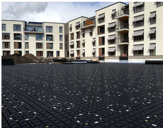
Blue-Green Roof Installation by Permavoid, Margeretha Gardens, Holland (credit: www.permavoid.co.uk )
