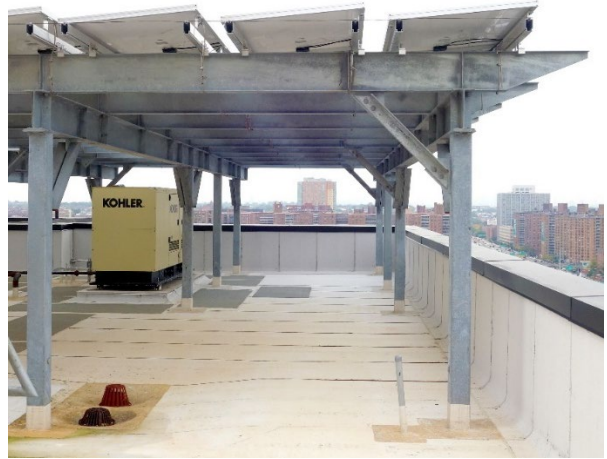
Concrete posts (left, credit: www.pvsolarfirst.com ) and steel posts (right, credit: FXCollaborative)
